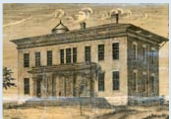
3 Berkshire Medical Institute 725 North Street
